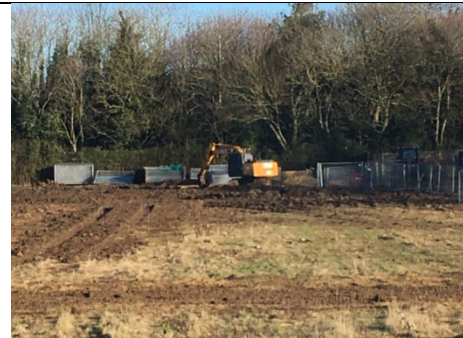
A lack of tree protection is evident, with extensive disturbance to ground by a digger within the protected RPA next to Chilton Priory boundary trees, in December 2019
